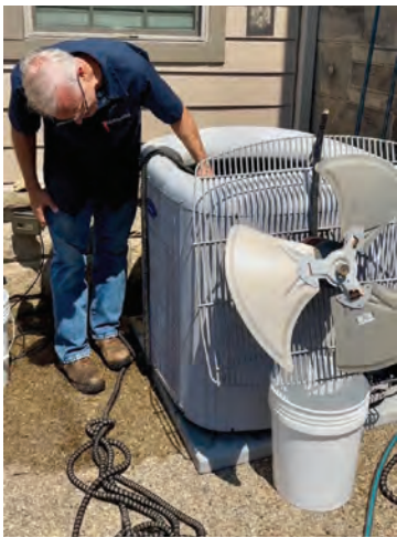
Dave Sienerth, Homelio technician performs routine maintenance on an air-conditioning unit. (Photo by Stacey Reibach)
